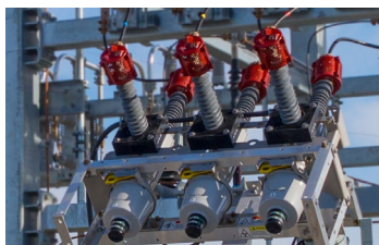
Viper-ST Recloser with one set of external CTs. A second set of CTs can be provided on the other side.
