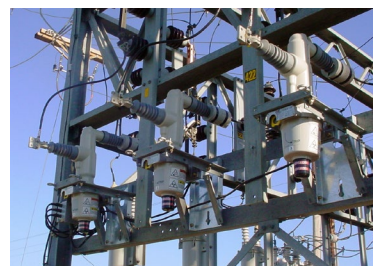
Retrofit installation with Z-shaped module Viper-ST Recloser on individual frames.
