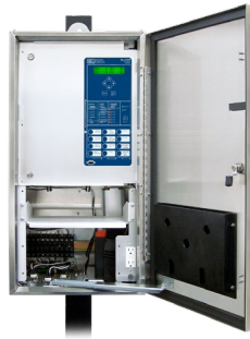
SEL-651R front access control for conventional recloser applications.
